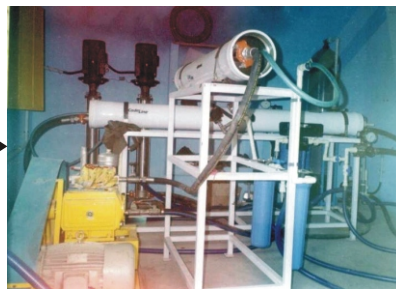
Synchronised 2-stage RO plant installed at Mullimunai village, Tamil Nadu
