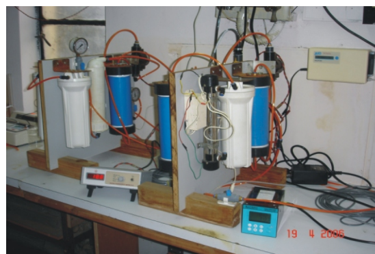
Ultrapure water production unit
