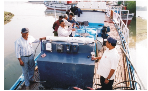
Barge mounted RO desalination unit installed in West Bengal
